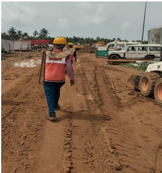
Job specific PPE (Hand gloves & Shoulder pad) using while engaged in steel bar shifting
