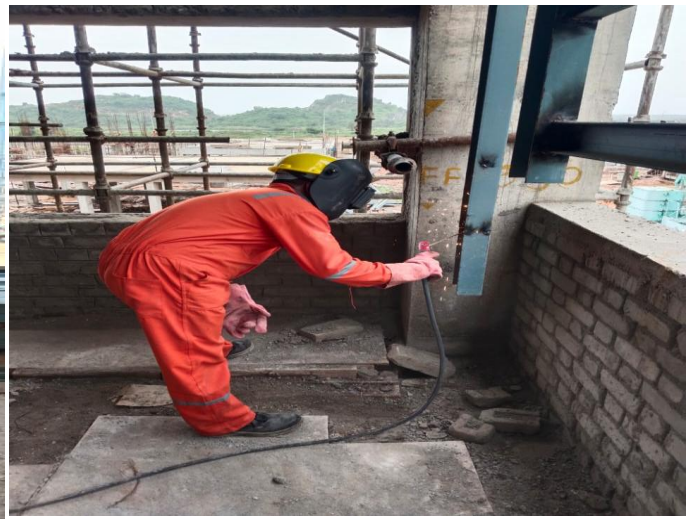
Job Specific PPE (Welding suit, Leg Guard, Face shield, Fire retardant gloves) used while performing Welding
