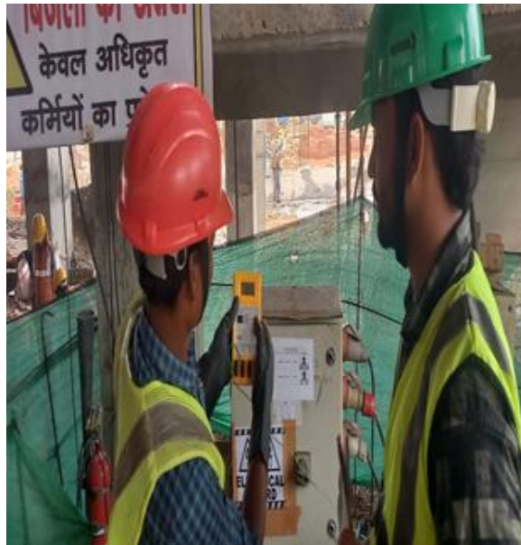
Job specific PPE (Rubber hand gloves) using while electrician performing electrical DB testing
