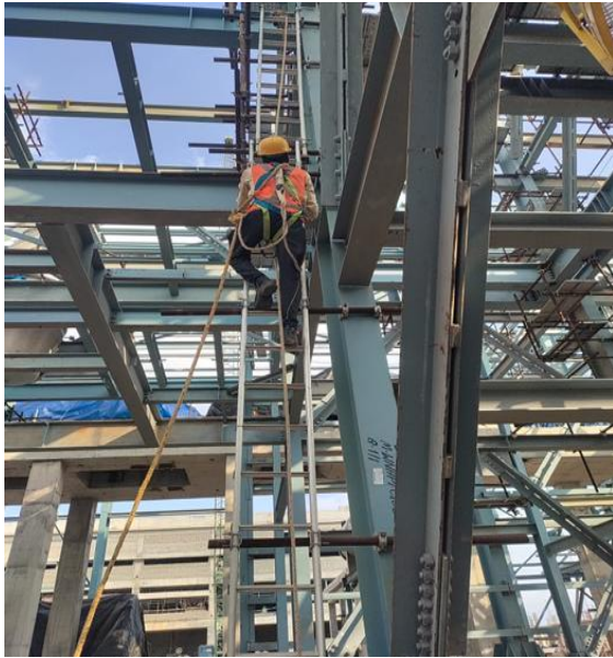
Job specific PPE (Full body Harness, Rope Grab) using while engaged in Height Work
