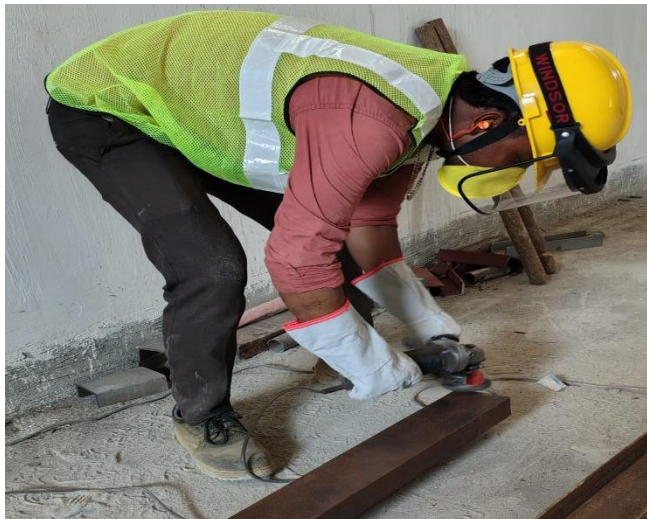
Job specific PPE (Hand gloves, Face shield, Ear plug) using while engaged in grinding job
